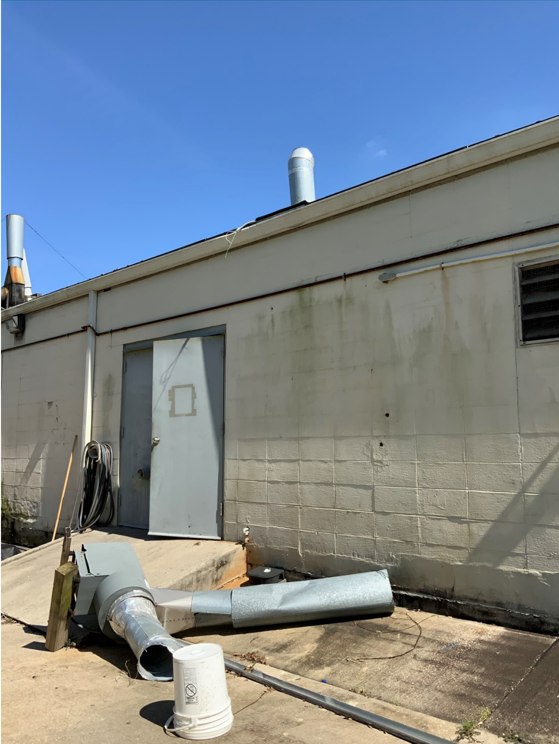
Figure E.5 – West Lab Maintenance (fan damaged during Hurricane IDA).
