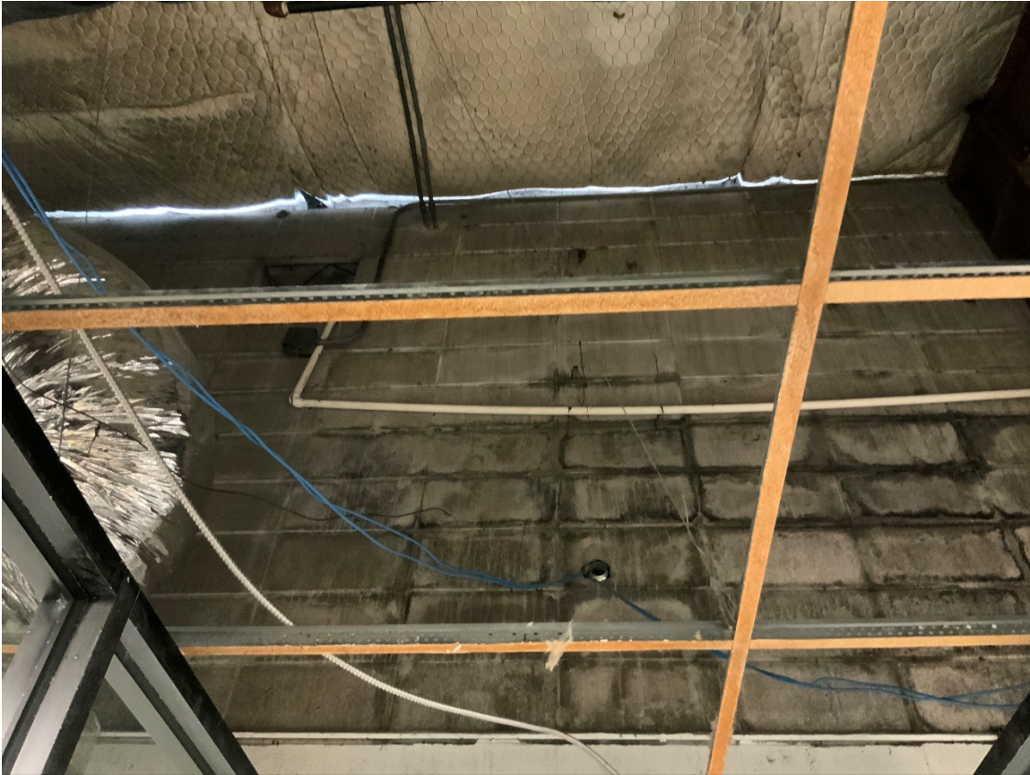
Figure E.1: West Lab Ceiling (where flashing removed due to Hurricane IDA).
